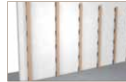
vertical support battening = installation CP horizontal
